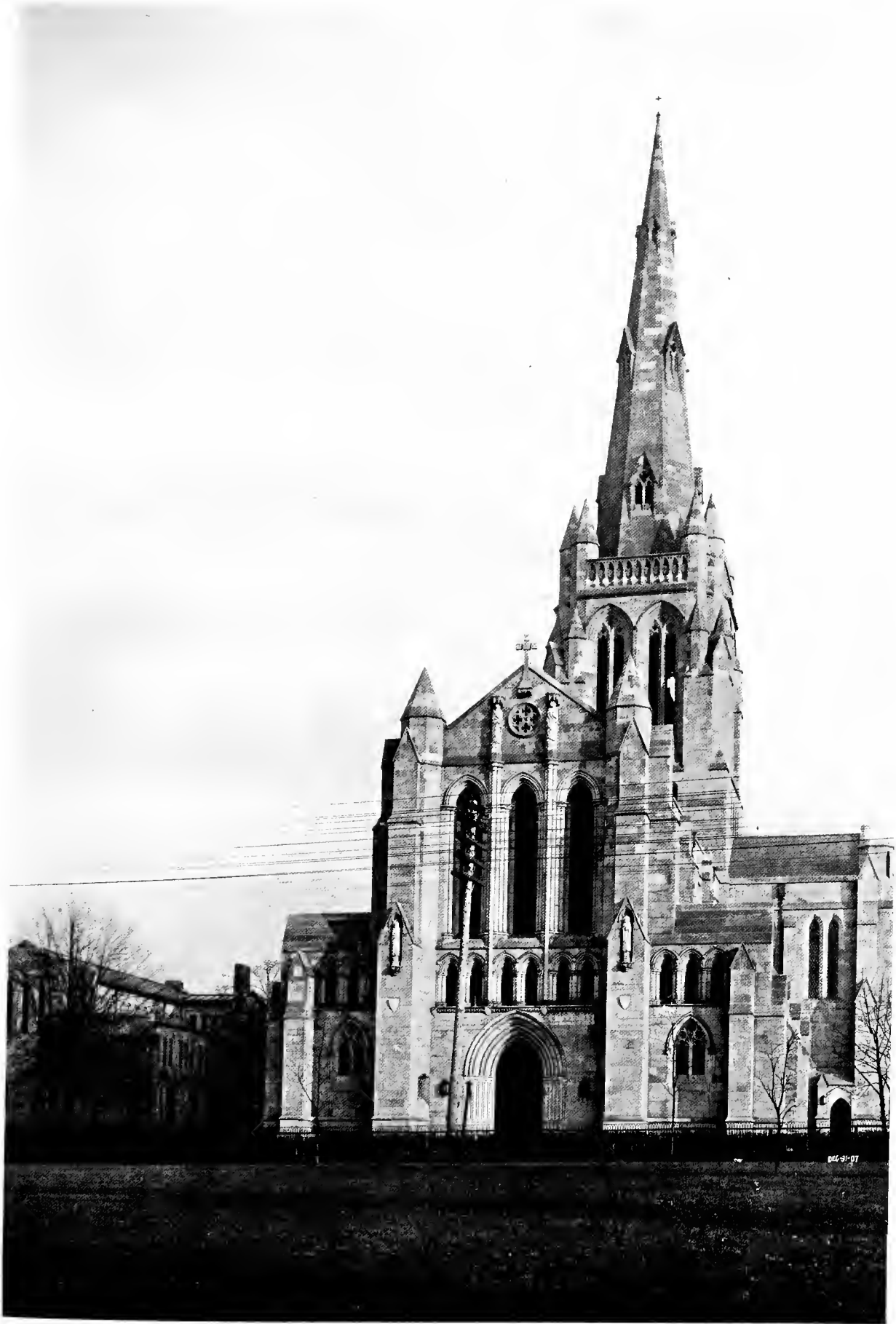
CALVARY CHURCH, PITTSBURGH, PA. MESSRS. CRAM, GOODHUE & FERGUSON (BOSTON OFFICE), ARCHITECTS
